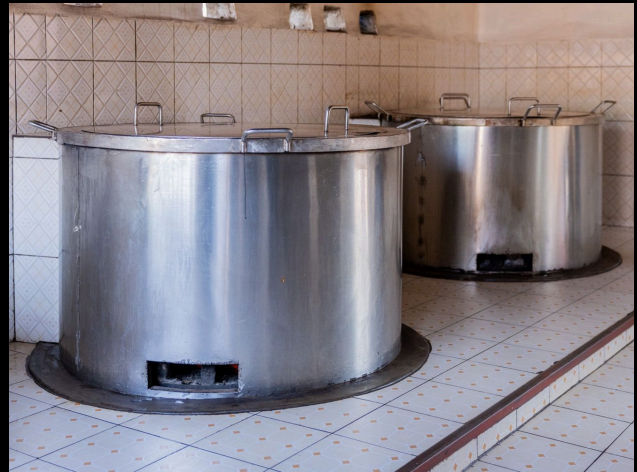
Energy-saving stoves in a school kitchen.
